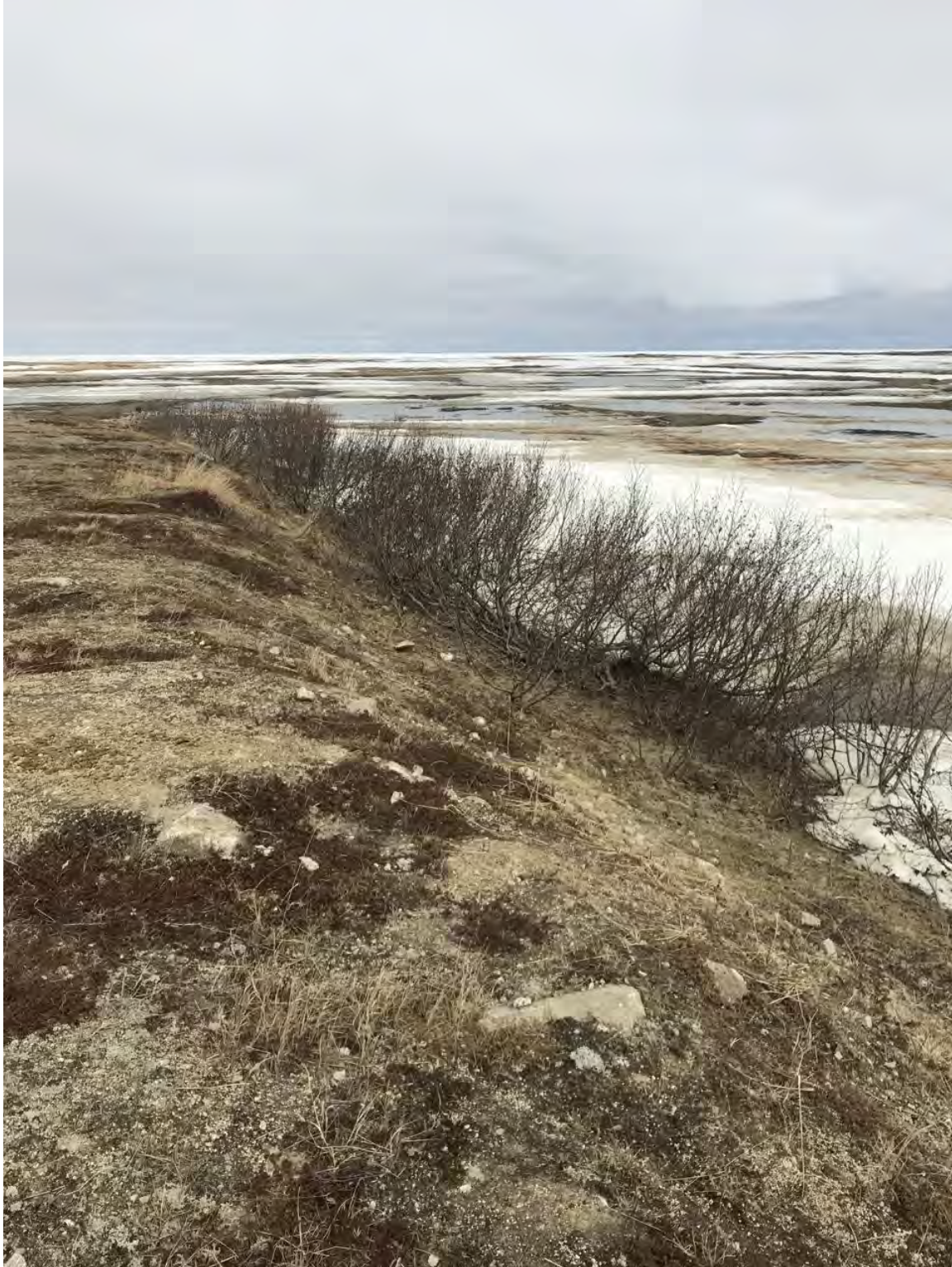
Figure 9. Side slopes at east terminal. Vegetation observed along bank with no obvious signs of scour or erosion from storms surge waves.
