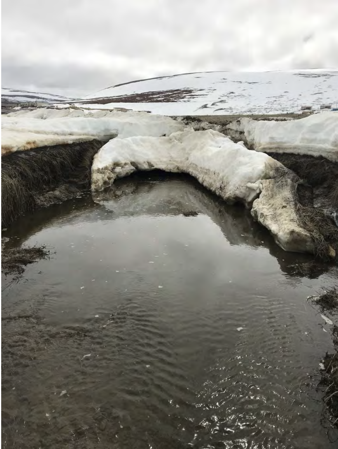
Figure 5. Runway culvert outlet.
