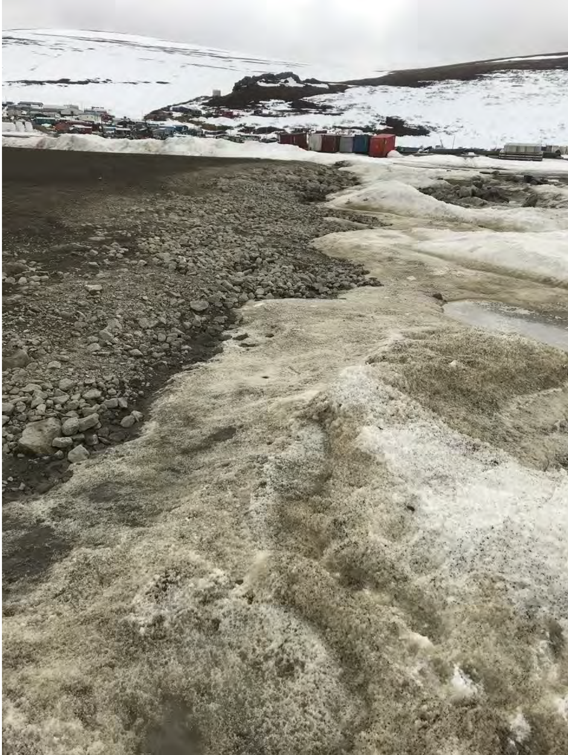
Figure 13. Western runway terminal. No armor rock observed.
