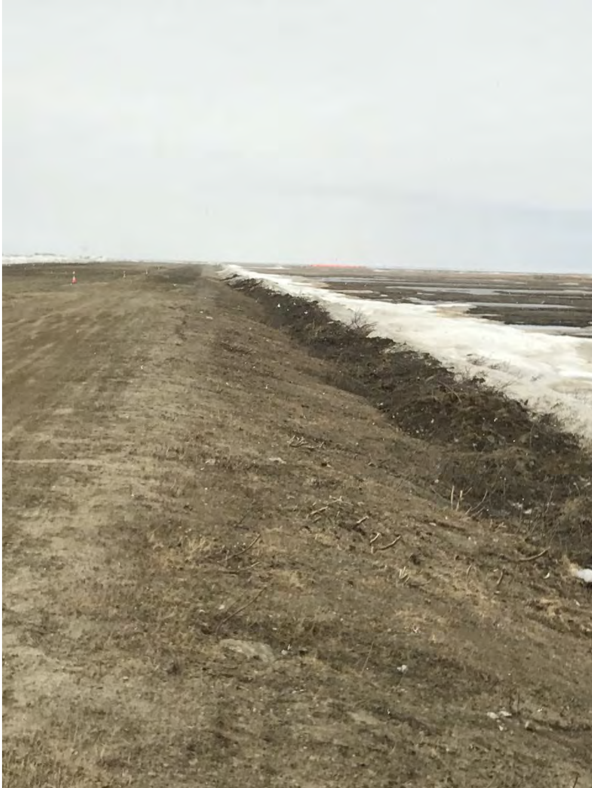
Figure 10. North slope of runway edge. No obvious signs of recent scour or erosion due to storm surge/waves (side slopes were noted to have been reworked/graded).
