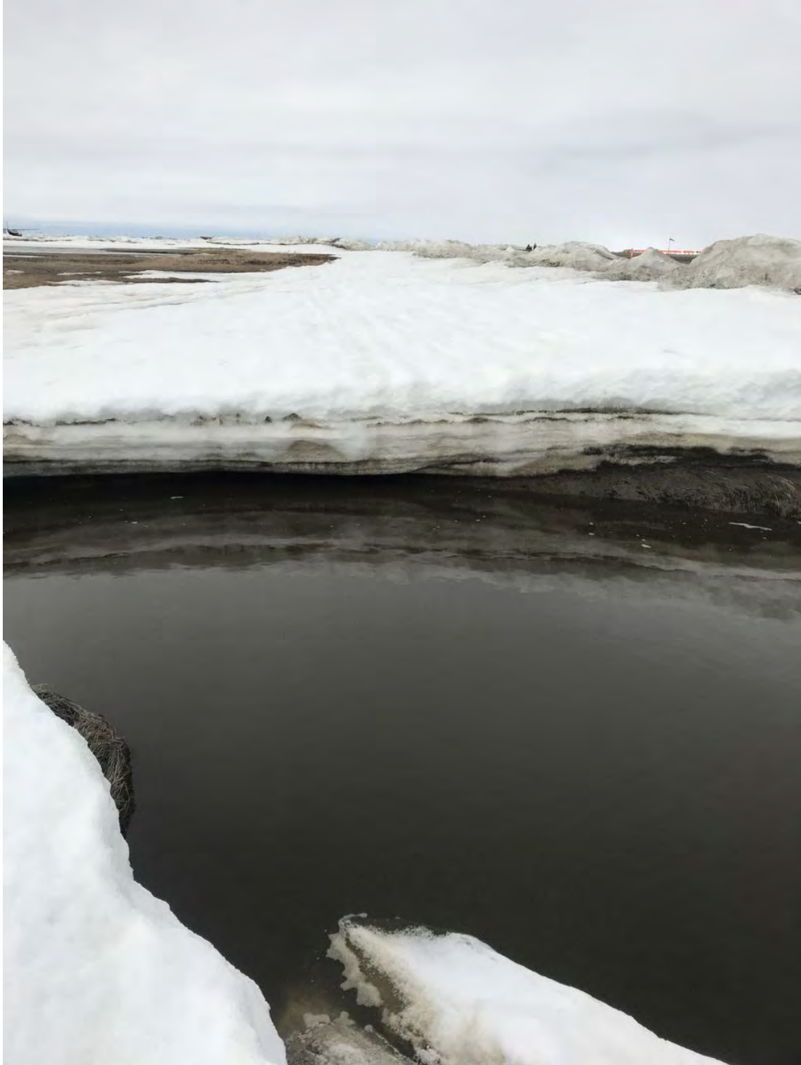
Figure 7. Pool at runway culvert inlet.
